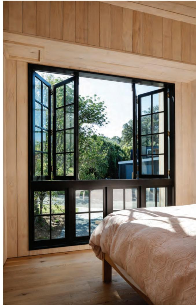
Materials and details are raw and unpretentious, detailed in familiar, low-tech timber construction. Band-sawn pine planks line the walls and ceiling, oiled cedar plywood and battens add a deeper colour on the back wall, and built-in seating maximises the use of space. The architect has avoided custom details to create a casual and relaxed atmosphere, with the only obvious 'city' elements being the plate steel balustrade and kitset steel kitchen by IMO.
