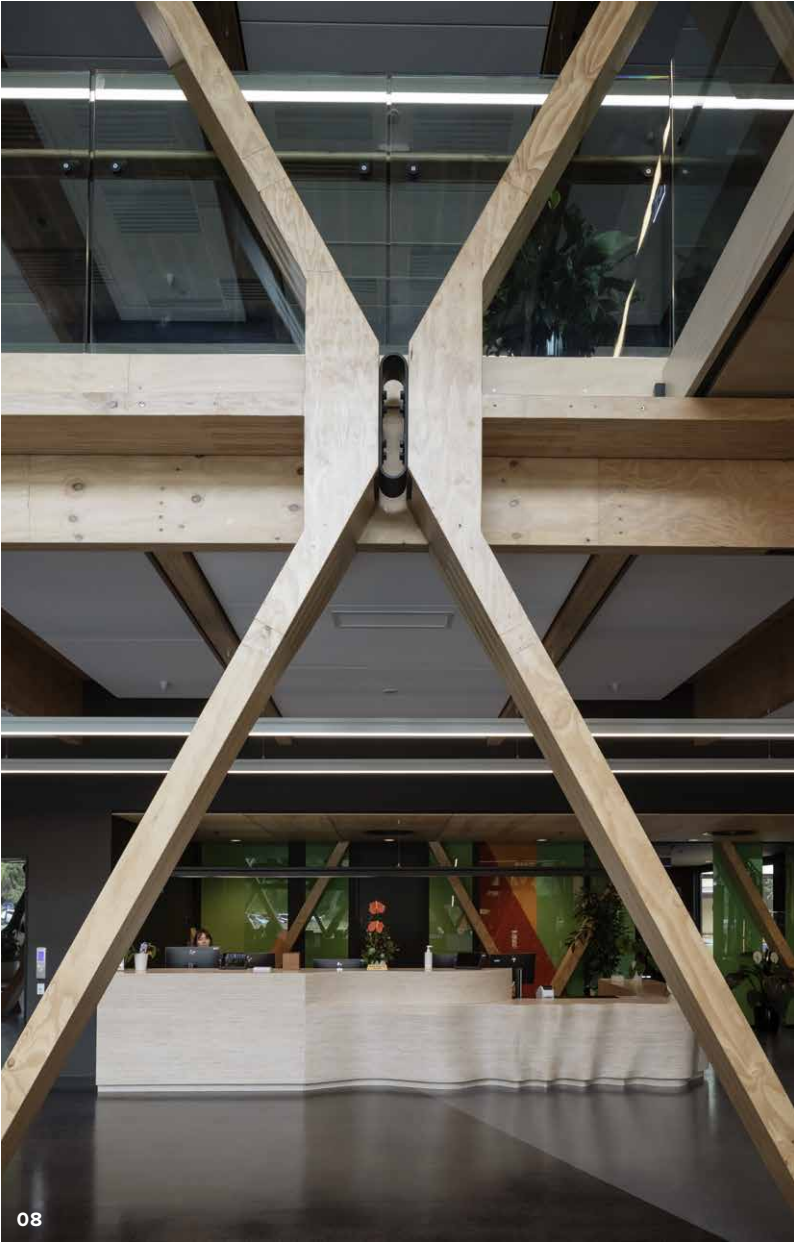
08 A U-shaped flexural plate (UFP), which acts as an energy-dissipation device between the diagrid elements. 09 The Hub makes a grand gesture at the heart of the campus, flanked by labs on either side.
